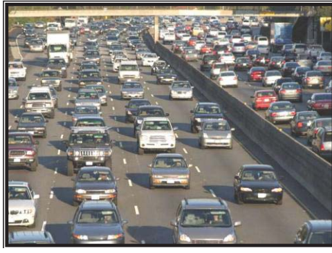
Level of Service F Driver Comfort: The Lowest Maximum Density: more than 67 passenger cars per mile per lane
