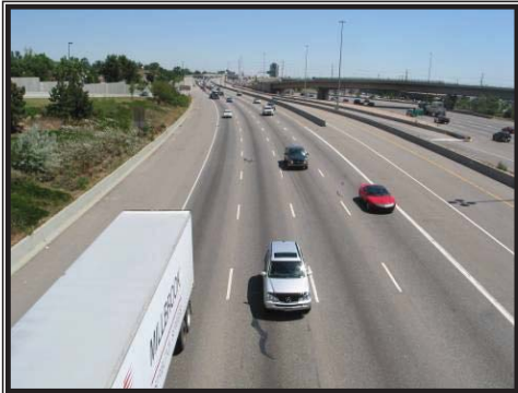
Level of Service A Driver Comfort: High Maximum Density: 12 passenger cars per mile per lane
