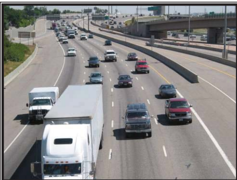
Level of Service C Driver Comfort: Some Tension Maximum Density: 30 passenger cars per mile per lane
