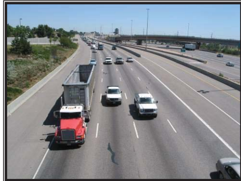
Level of Service B Driver Comfort: High Maximum Density: 20 passenger cars per mile per lane
