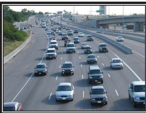
Level of Service E Driver Comfort: Extremely Poor Maximum Density: 67 passenger cars per mile per lane
