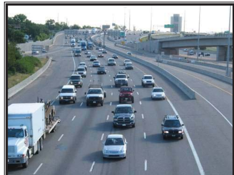
Level of Service D Driver Comfort: Poor Maximum Density: 42 passenger cars per mile per lane
