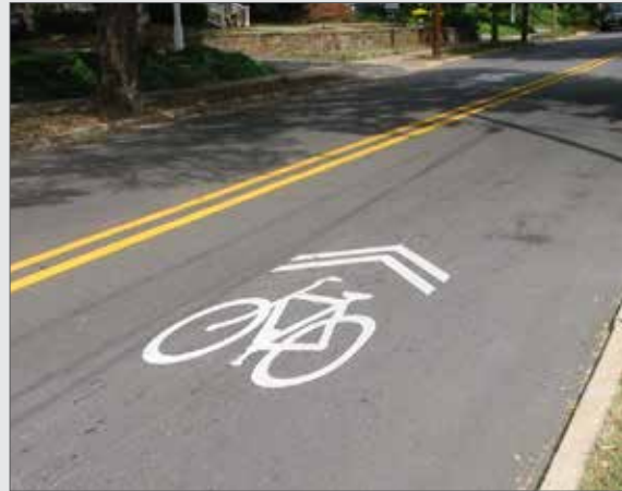
Example of shared-lane markings on pavement.
