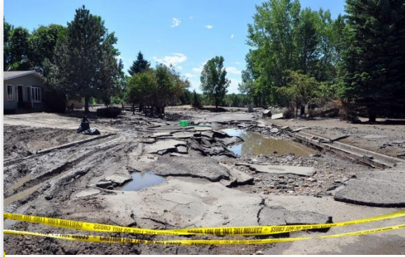
Category C Roads and Bridges
