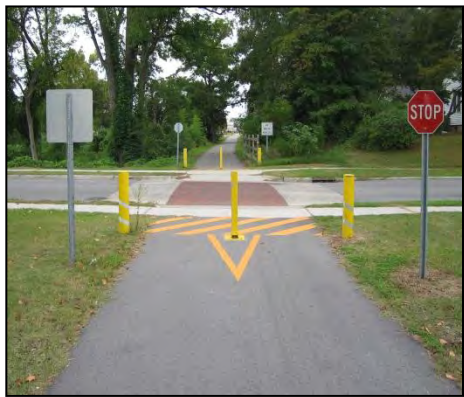
A raised speed table and trail crossing in Williamston, NC. Photo courtesy of Rivers & Associates, Inc.
