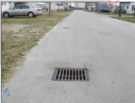
Drainage grates with wide openings can become hazardous for bicyclists. Photo Courtesy of Rivers & Associates, Inc.
