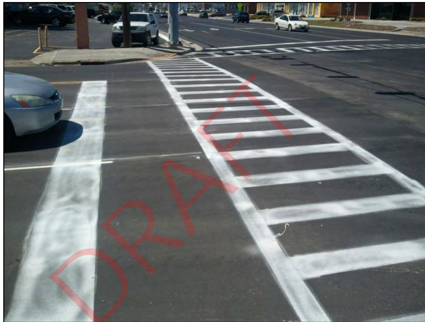
Hybrid standard/ high-visibility crosswalks under construction at the NC 58 and Atlantic Beach Causeway intersection. Photo Courtesy of NCDOT.
