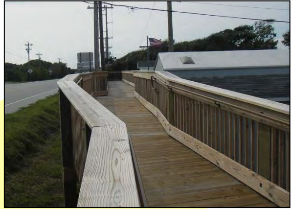
The existing boardwalks located near the Atlantic Beach / Pine Knoll Shores town limit is too narrow to accommodate bi-direction bicycle traffic. Photo courtesy of Rivers & Associates, Inc.
