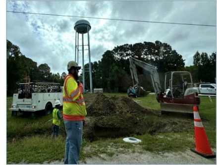
Water system work underway this morning – photo taken on Broad St:
